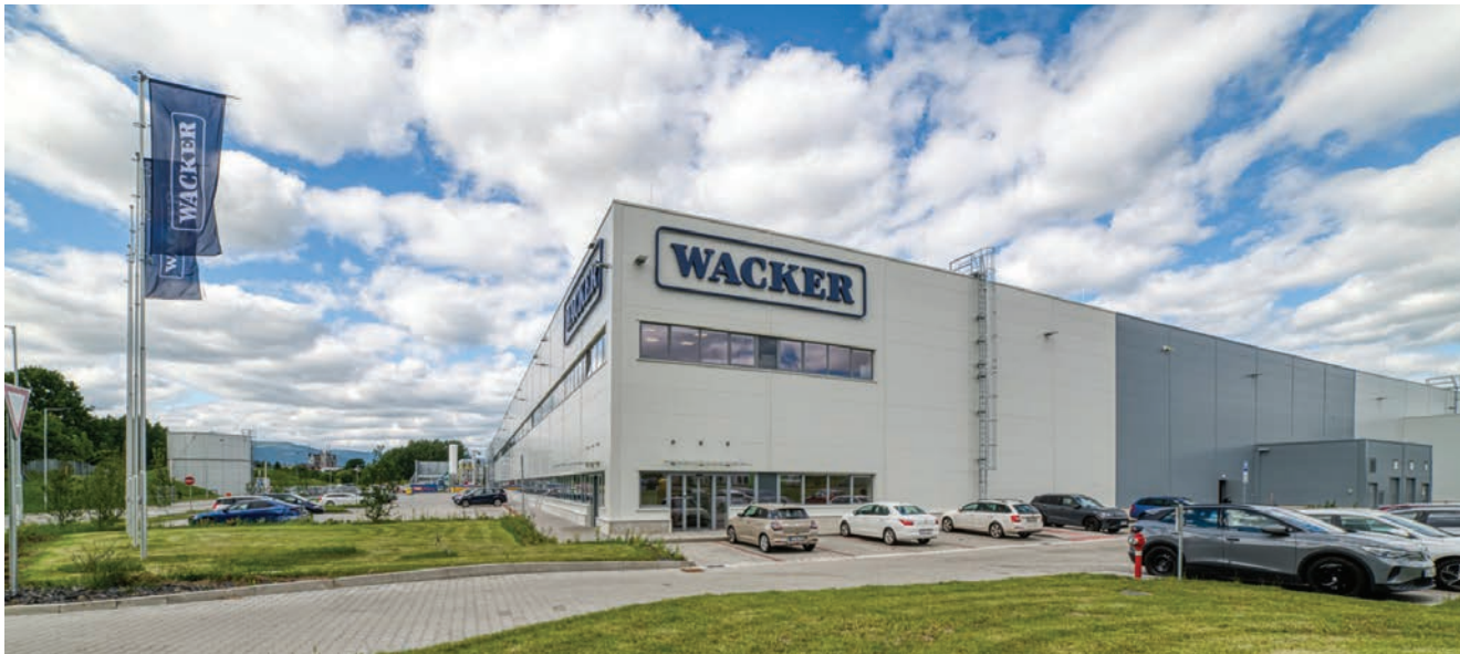
At WACKER's new Czech based production site in Karlovy Vary, WACKER will produce silicones for the growth markets of electromobility, medical technology and power-grid expansion. Source: WACKER
