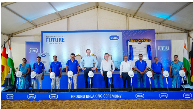
Leadership team breaking ground at the future R. STAHL facility in Sriperumbudur SEZ
