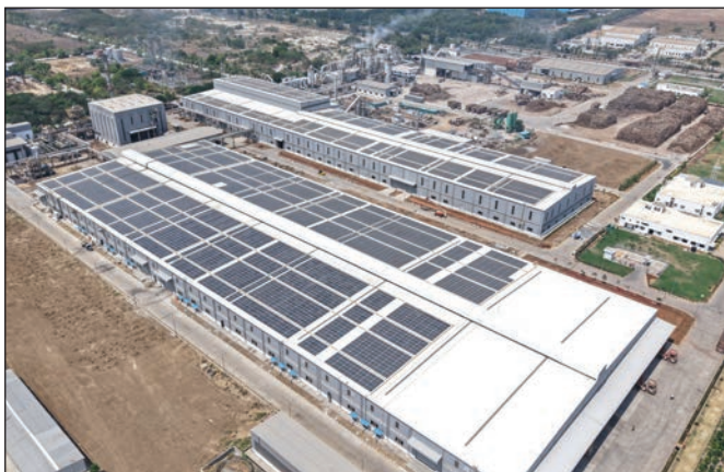
Roofsol Energy Project: Greenlam Industries Ltd, Naidupeta, Andhra Pradesh, 4MWp
