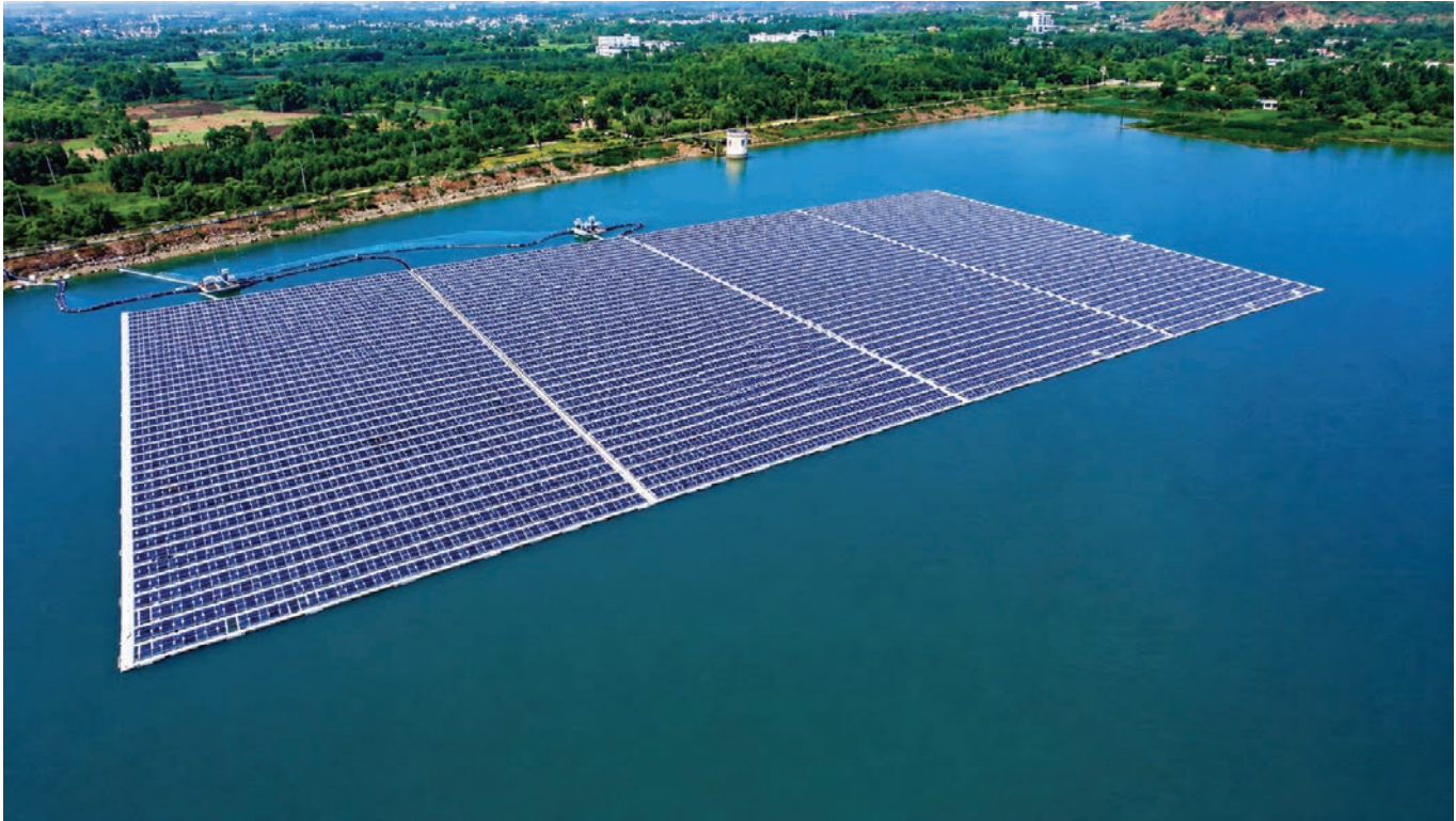
TrueRE's floating solar project, Visakhapatnam, Andhra Pradesh
