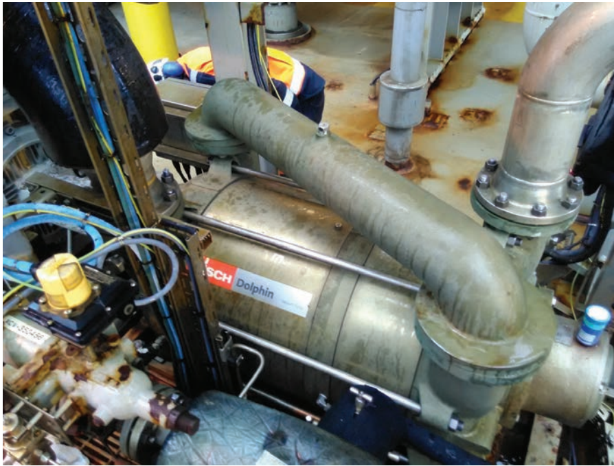
A DOLPHIN liquid ring vacuum pump from Busch Vacuum Solutions. Source: Busch Vacuum Solutions.
