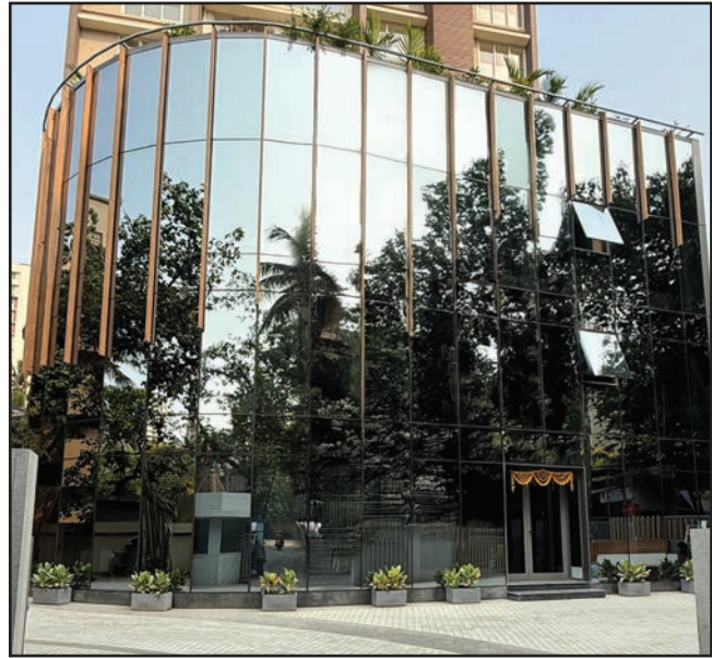
Current CPP office in Mumbai.
