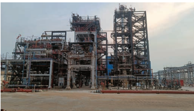
Figure 4: Second commercial indJet® unit at IndianOil refinery.
