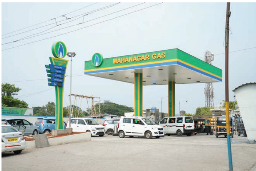
Mahanagar Gas Limited CNG station
