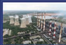
Lignite based Power Generation 3640 MW
