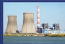
Coal based Power Generation 1000 MW
