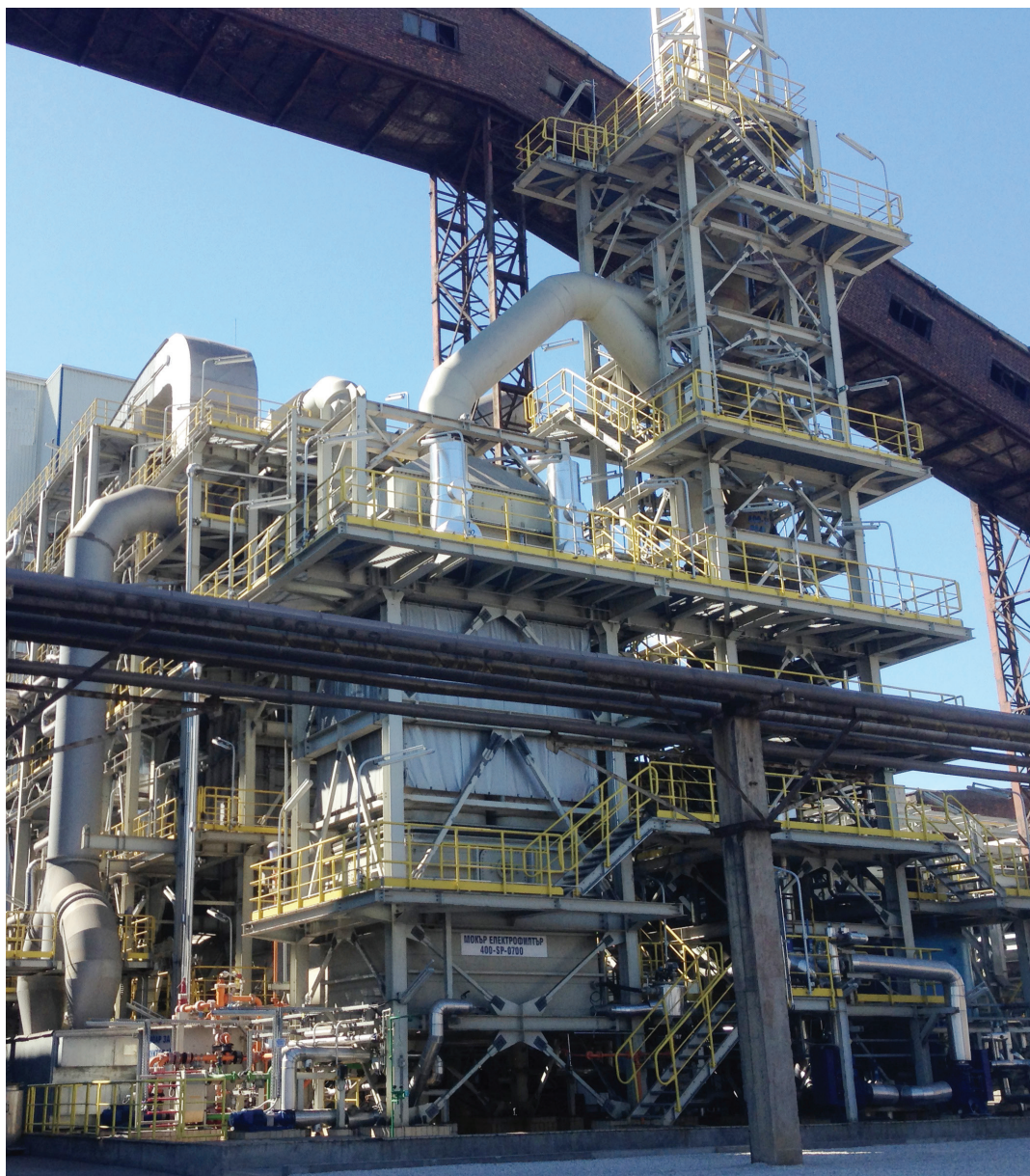
OXYSULF Wet Sulfuric Acid Plant
