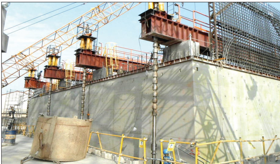
Figures 5 : Pushdown Caisson using ground anchors and computerized jacking system
