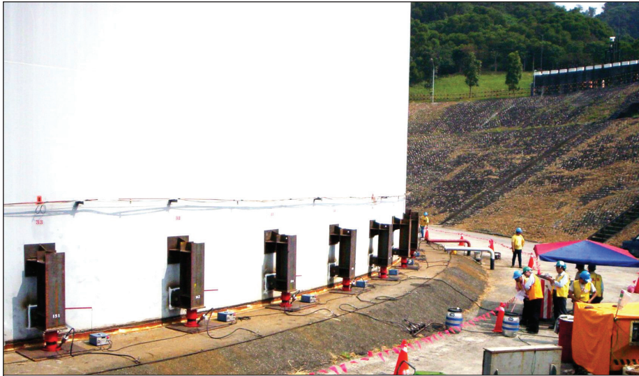
Figures 3 : Renovation of storage tank by using intelligent structure jacking system
