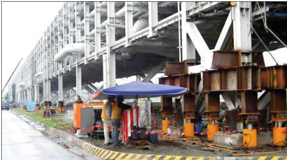
Figures 4 : Extend Pipe Rack service life by using computerized jacking system
