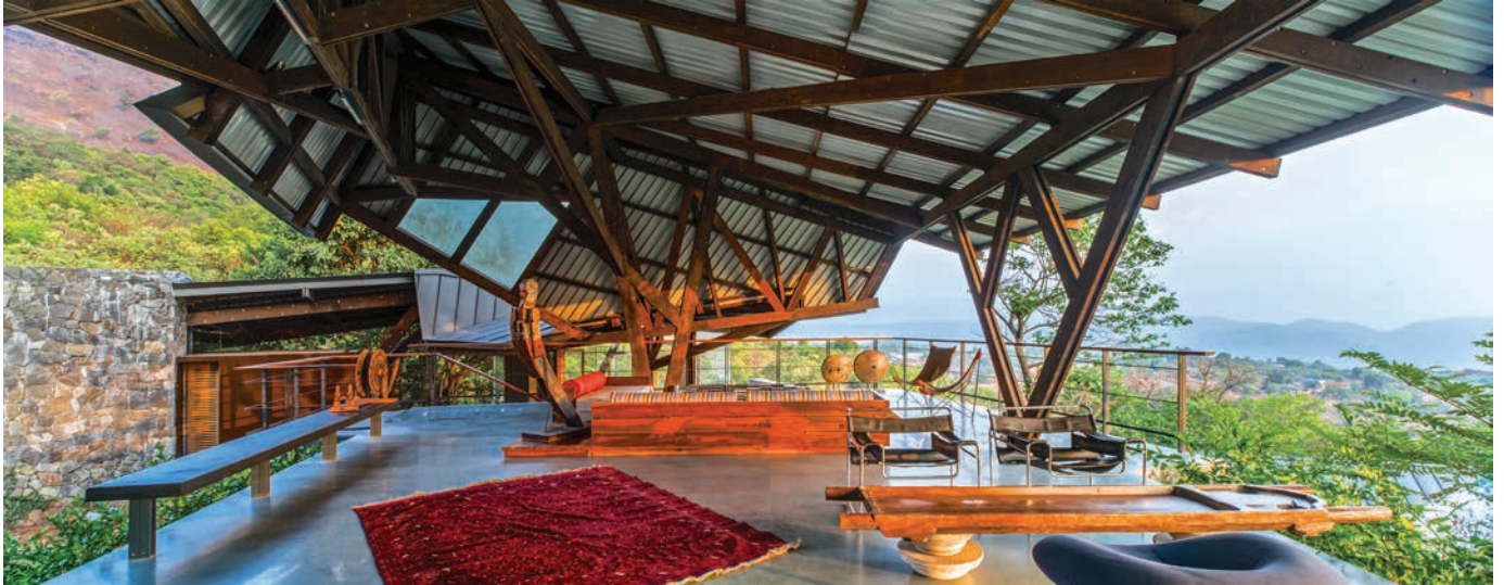
A composite structural tree-like truss section shades the outdoor living area.
