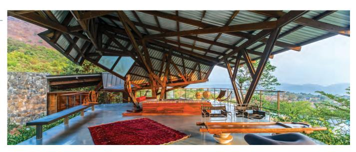
A composite structural tree-like truss section shades the outdoor living area.
