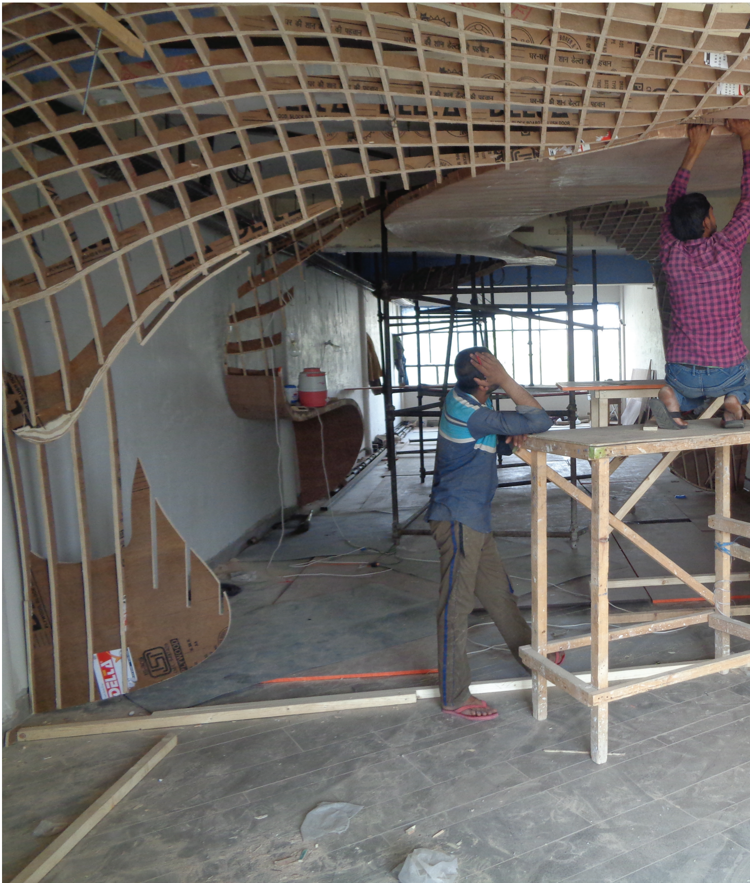
The ribs were jig-sawed in-situ, by the carpenters, in a unidirectional arrangement to correctly align to the next segment.
