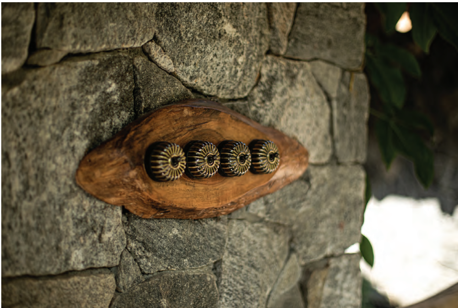
Up-cycled wood from site is repurposed into switchboards while retaining its organic shape.
