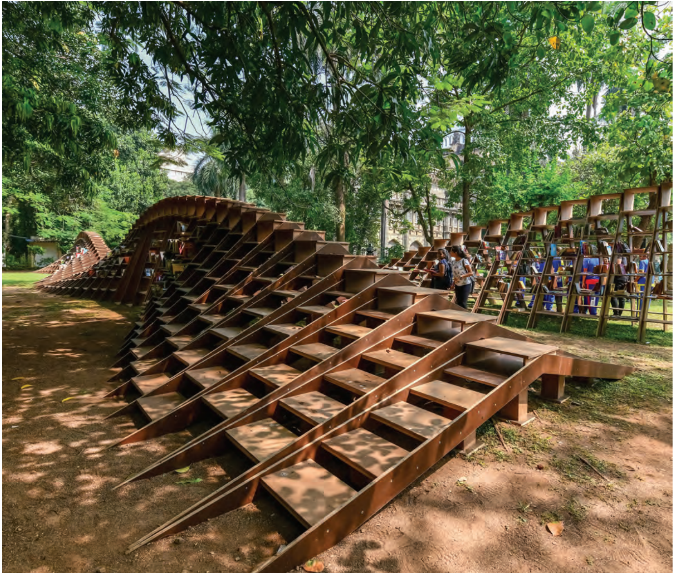
3,600 modular pre-fabricated components were used to construct the 'worms.'
