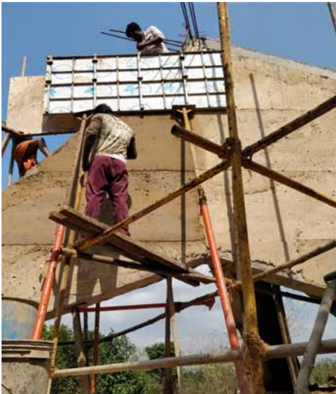
↑ Fixing the shutters.
