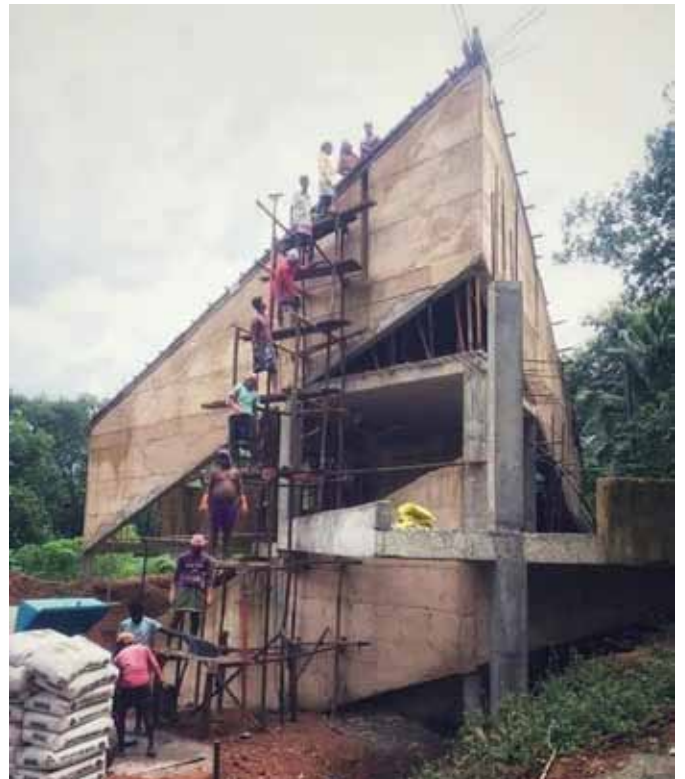
↑ Roof slab concreting.
