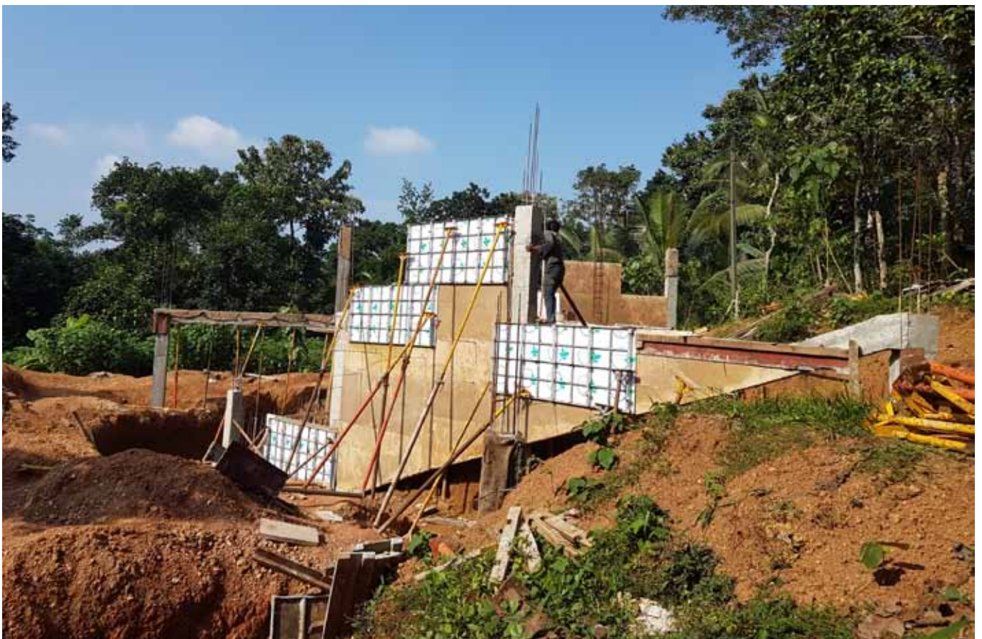
↑ The shuttered debris wall in progress.
