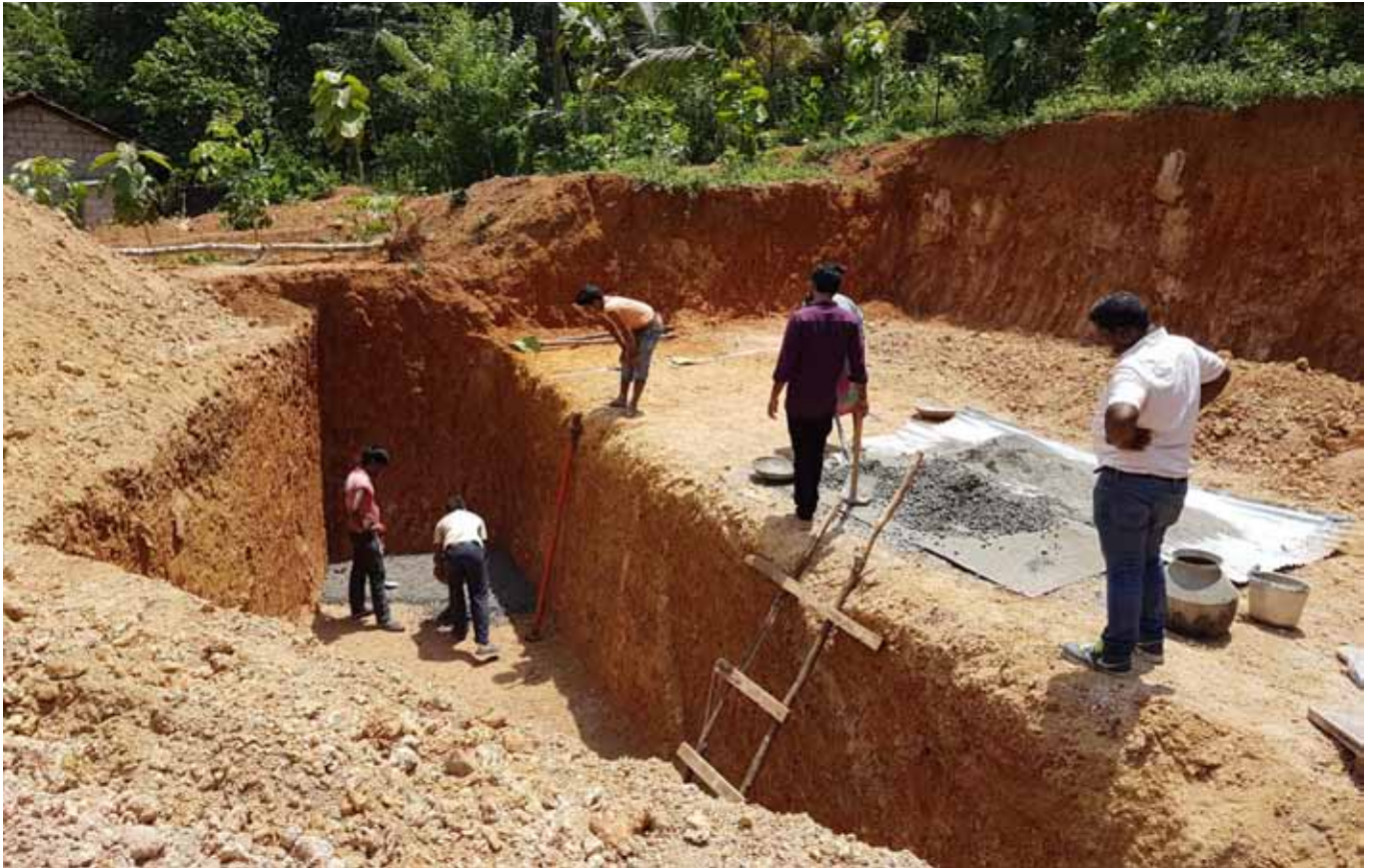
↑ Rainwater Pit: The excavated soil was used for shuttered debris wall.
