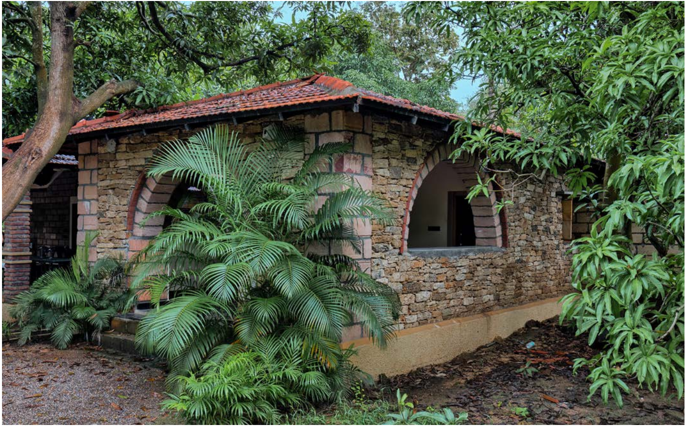
The construction harks back to traditional techniques like sandstone arches and random rubble walls.
