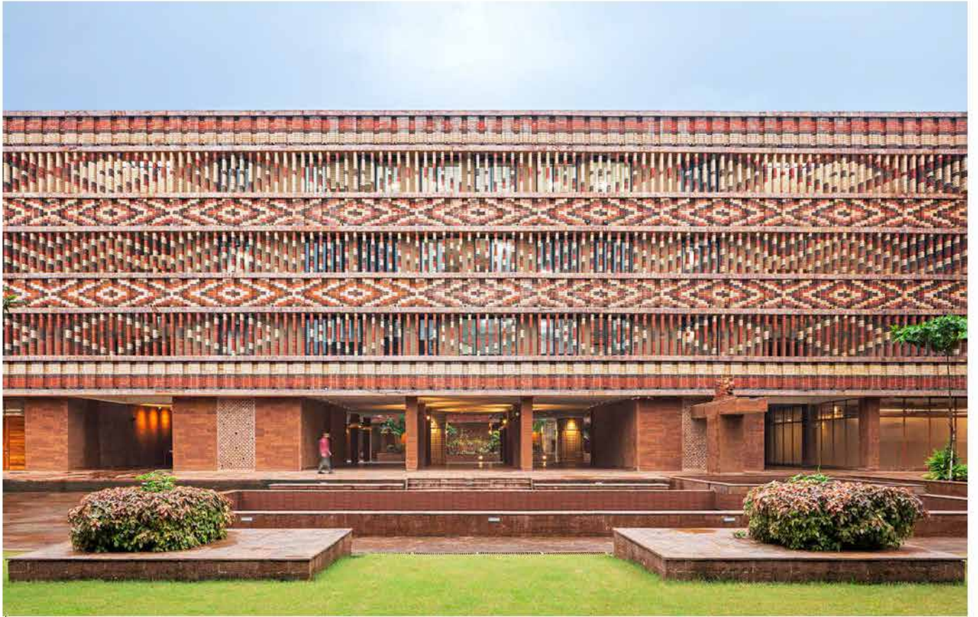
† The upper floors of Krushi Bhawan feature a distinctive brick façade inspired by Ikat patterns of Odisha handlooms, created using clay in three different colours.
