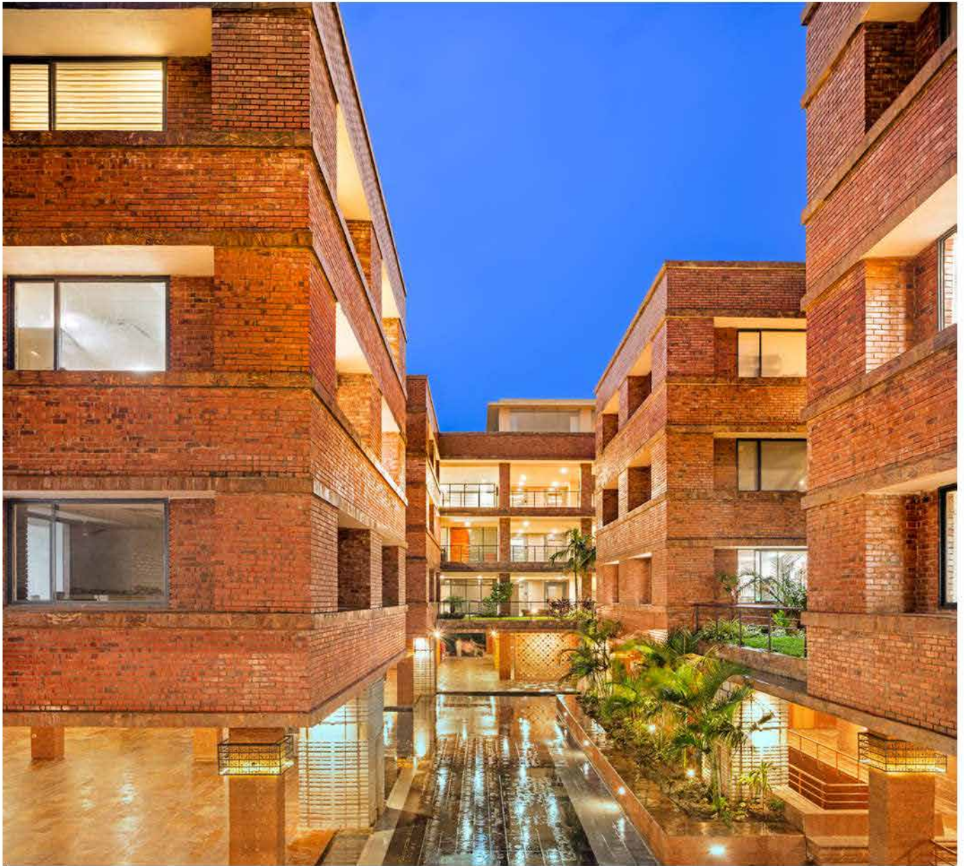
† The building achieves high thermal comfort for its users while cutting down the need for air-conditioning via HVAC systems to only 20% of the built spaces.
