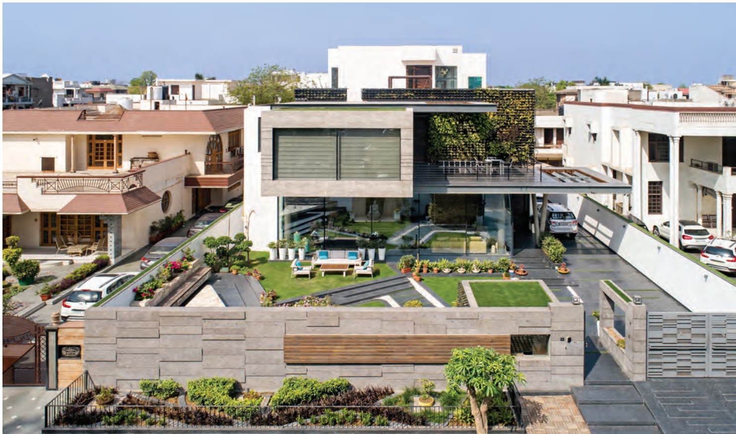
The master bedroom, located on the first floor is designed as a cantilevered block to break the mass of the house.
