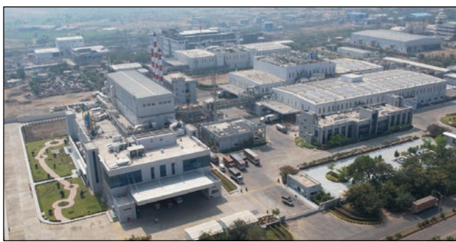
Henkel Adhesive Technologies' Kurkumbh facility.
