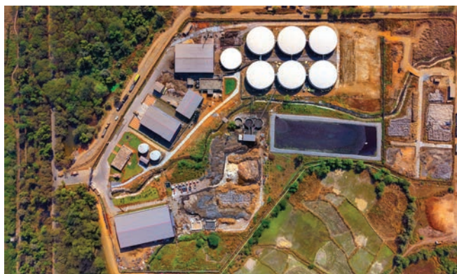
India's fastest CBG plant to achieve 21+ TPD capacity
