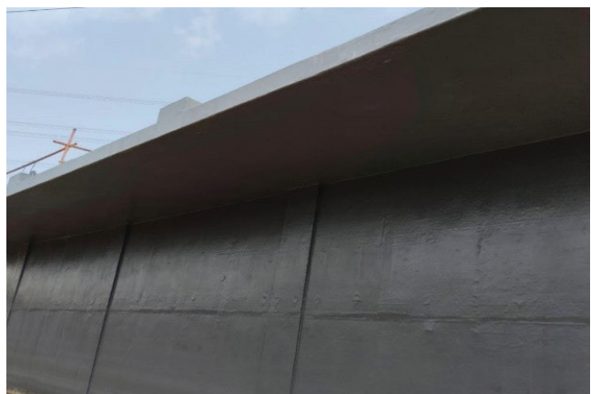
FRP lining to Aeration basin.
