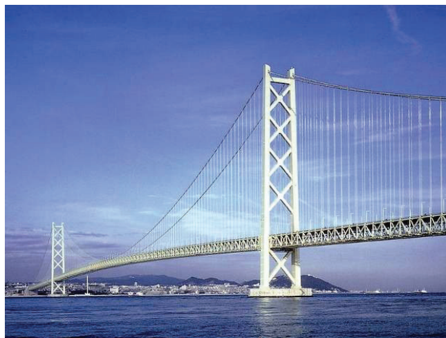
Fig 2: Honshu-Shikoku Bridge, Japan coated with CORRPASSIVE, conductive polymer based coating system
