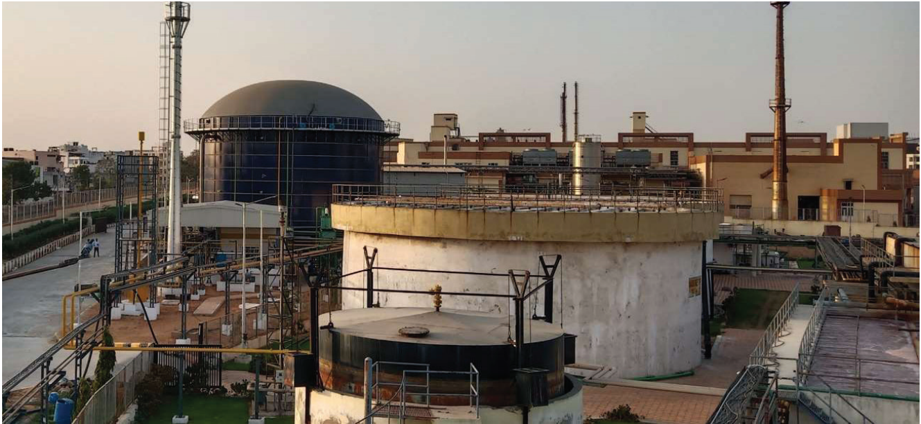
Overview of sludge management plant
