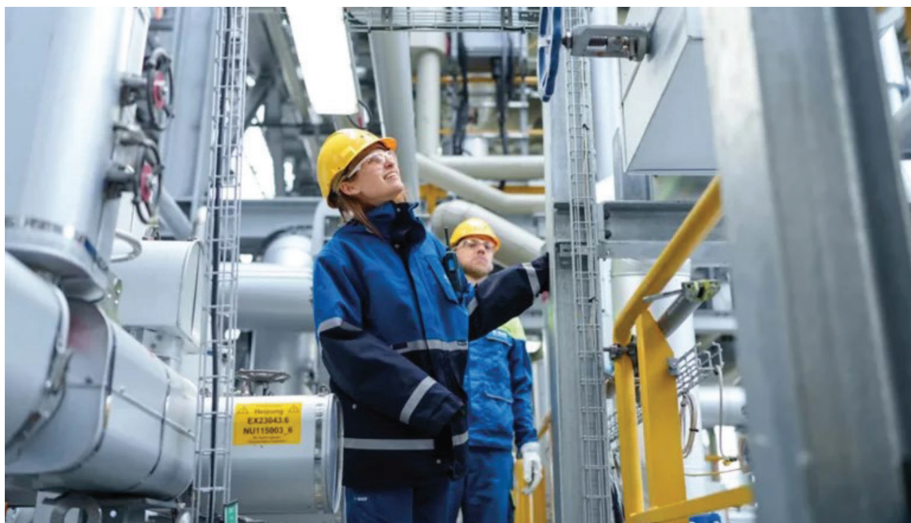
E-Furnace Demonstration Plant at BASF's Ludwigshafen site
