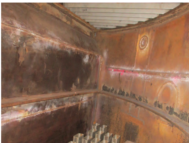
Figure 3: New Dividing Wall Inside RFU Splitter II
