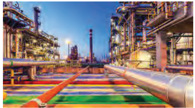
MOL Group Downstream Facility (Pic Courtesy: MOL Group)
