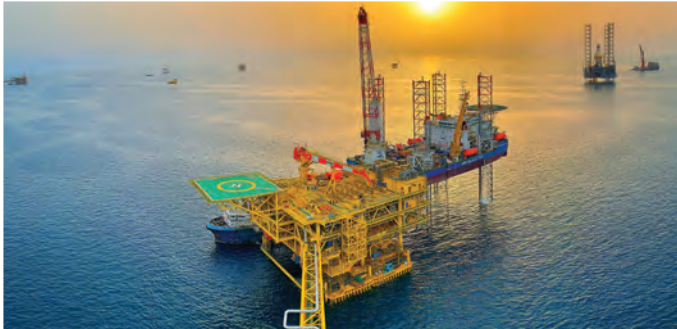
A fully integrated gas platform installed by float-over method at the Hasbah field in Saudi Arabia
