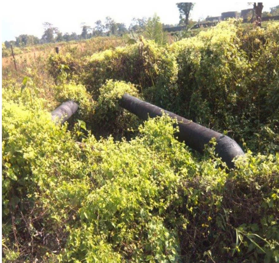
Figure 4: Complex network and difficult to navigate right of way
