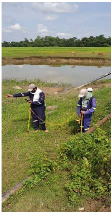
Figure 5: IIIT survey of XLI being performed for OIL pipeline network
