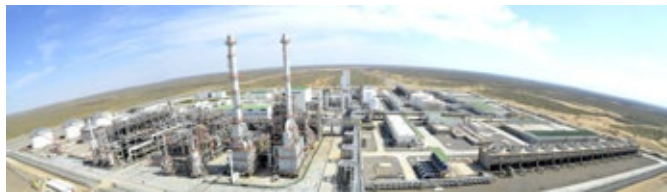
The world's only large-scale natural gas-to-gasoline plant produces 15,500 barrels-per-day of gasoline. Nacero's planned facility will have more than double that capacity.
